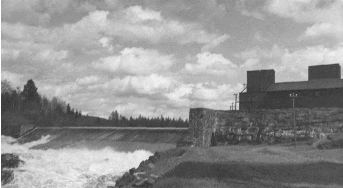
Gravity dam and "Bulk Head" - Source: City of Shannon archives
