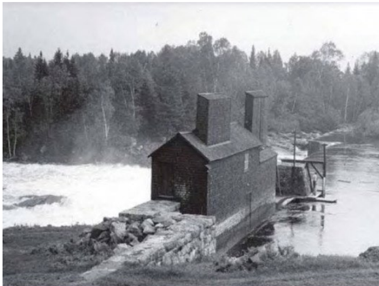
“Bulk Head” and gravity dam – Source: City of Shannon archives
